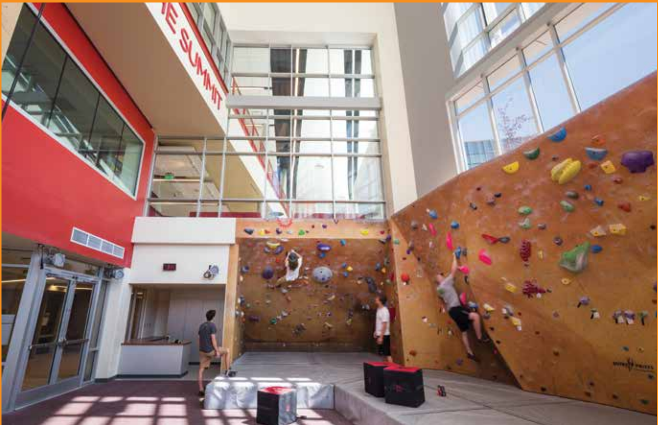
Left: 60-minute doors and storefront window with butt joint glazing Center: 60-minute curtainwall Right: Non-rated curtainwall
